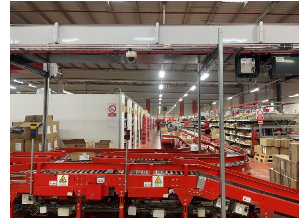
Würth factory with Telefonica solution deployed
